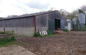
I) Steel-framed covered silo, 75' x 30'. Spaced boarding gale cladding with box profile side cladding above mass concrete wall.
