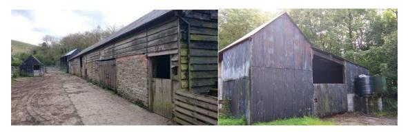
F) Redundant Concrete-framed Fodder Store in 5 bays, asbestos cement roof. The sheep dipping bath located to the south of the building and all associated equipment is also redundant.
